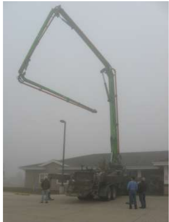
Stretching his arm over our building to pour concrete
