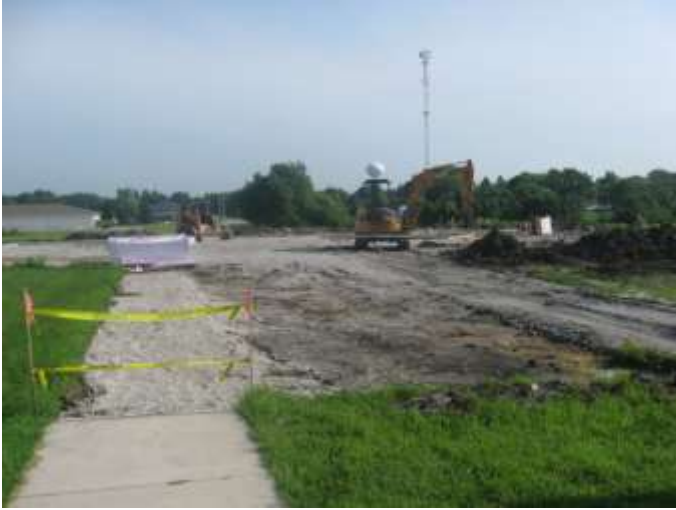
Breaking ground and leveling things off
