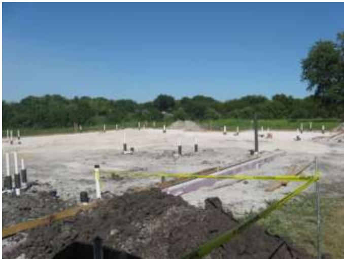
Plumbing pipes ready
